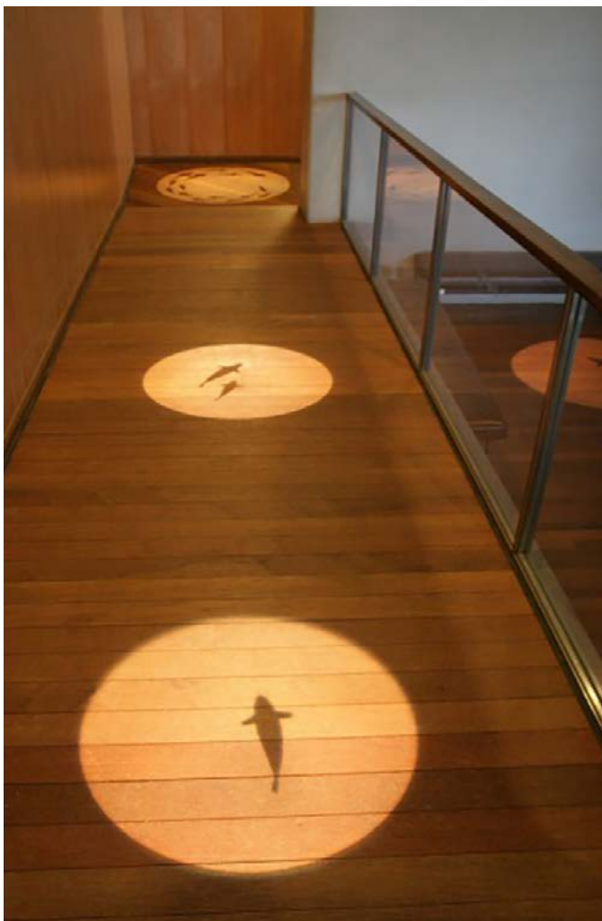
Grand Lighting GL10C4 Downlight with custom B&W Glass Gobos
